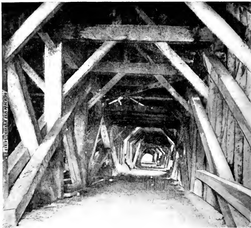
Interior of the Bridge.
